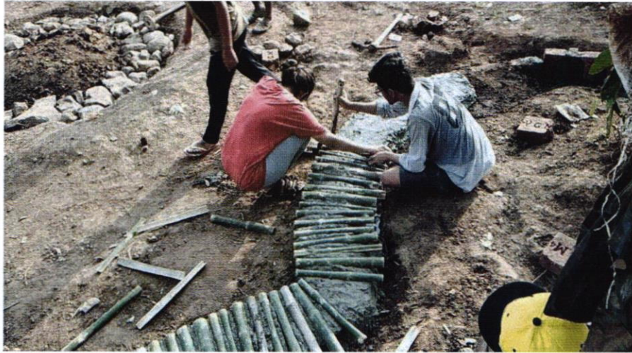
Students creating the foundation for the final structure
