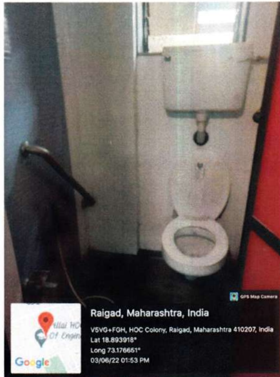
WASHROOM FOR DIVYANGJAN
