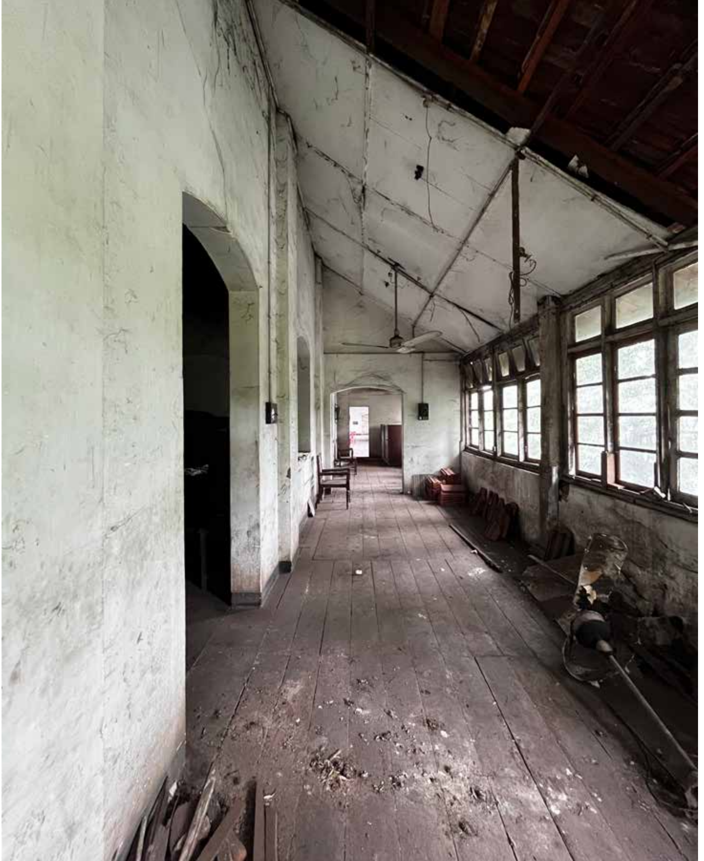
The floors of the first floor are paved in wood; ceiling was recently added under the tile roofs.
