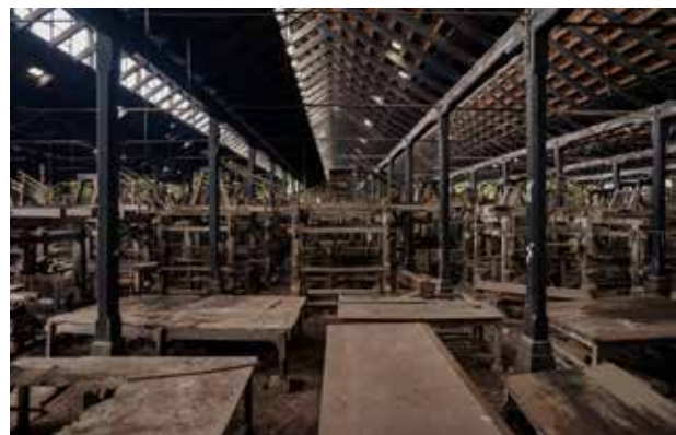
The weaving looms of the factory is in the hall that has a beautiful north lighting system. The looms have been ruined over the years. The columns are made of wood and joined using metal bolts.
