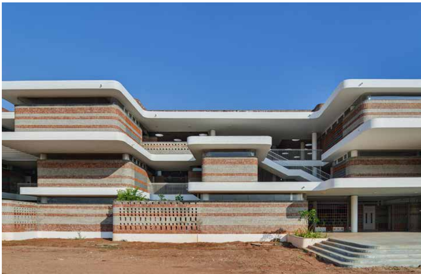
Structural system has been integrated in such a way that no columns are visible in the facade
