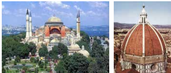
The Hagia Sofia Istanbul and Duomo Florence . Both Show ingenious approaches to creating wide span structures and offer insightful lessons
