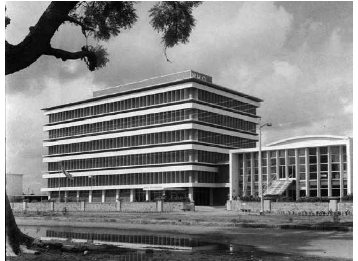
W.H.O Office building, New Delhi (Source: https://www.re-thinkingthefuture.com )
