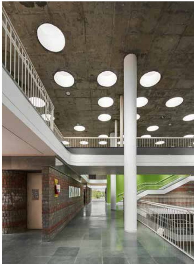
Circular glass openings in the ceiling bring in natural light into the courtyard
