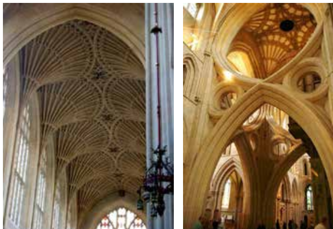
The Fan vaulting Oxford Chapel , Scissors arches( Wells Cathedral) are e.g.. of structure as Architecture in the medieval period.
