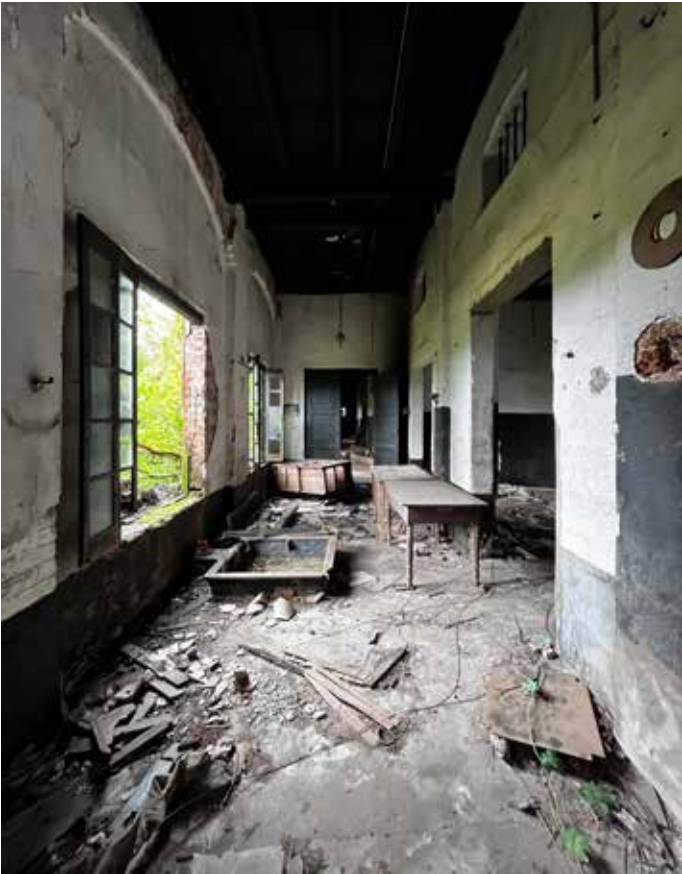
Condition of the south wall of the main building.
