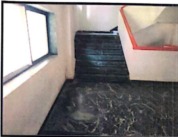
Daylight at Staircase
