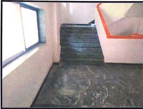
Daylight at Staircase
